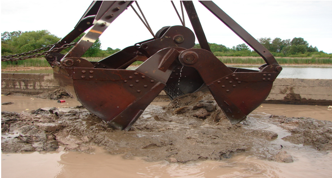
A clamshell bucket unloads sediment onto a barge
