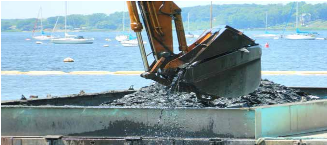
Unloading contaminated sediment onto a barge
