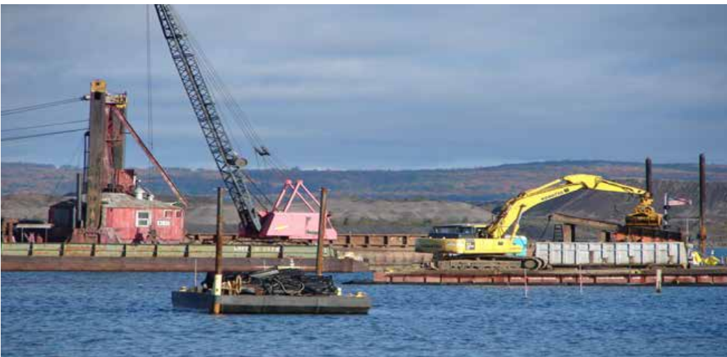
Environmental dredging in River
