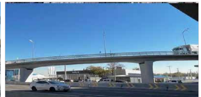
Post-tensioned interchange legs
